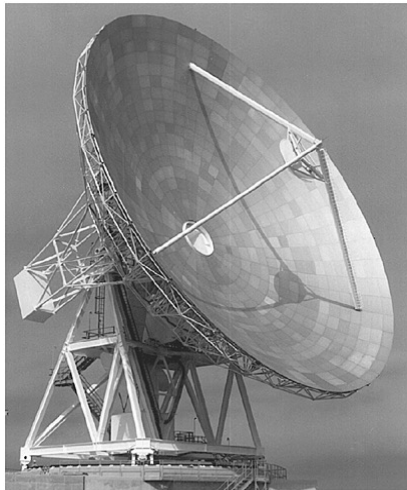
Class A earth station
