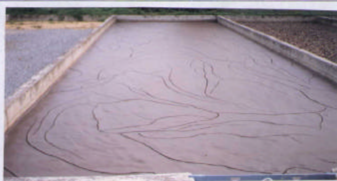
3. Next it is released again into large tanks filled with layers of sand and metal for the water to be removed down under the ground which flows into the near by river.
