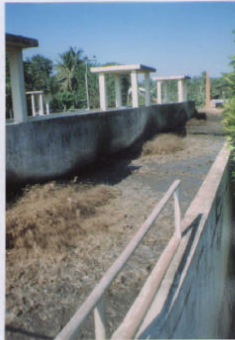
2 Then goes up through the three pipes into large tanks for stirring up with chemicals added.
