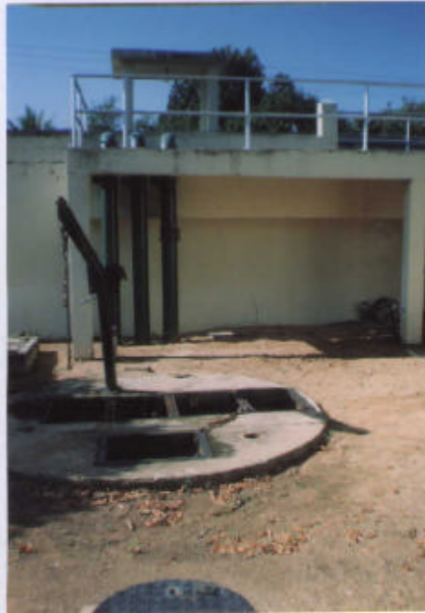
No :1 The well to which about 200 cubic ft of liquid solid waste gathers daily
