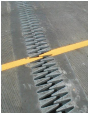
Figure 1.1: Thermal expansion joints in a roadway.
