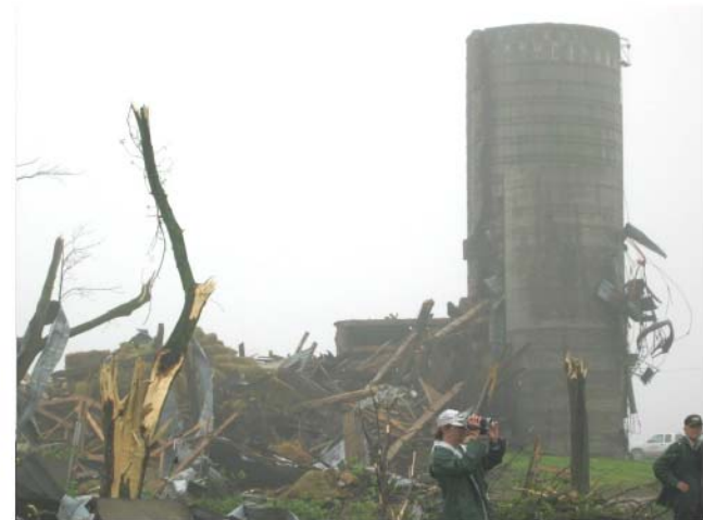
Example of SBO DOD8 with barn (at centre) completely destroyed (2004 Gad's Hill tornado)
