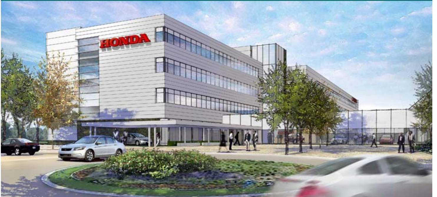
Honda Canada headquarters is currently under construction in Markham. Source: HOK
