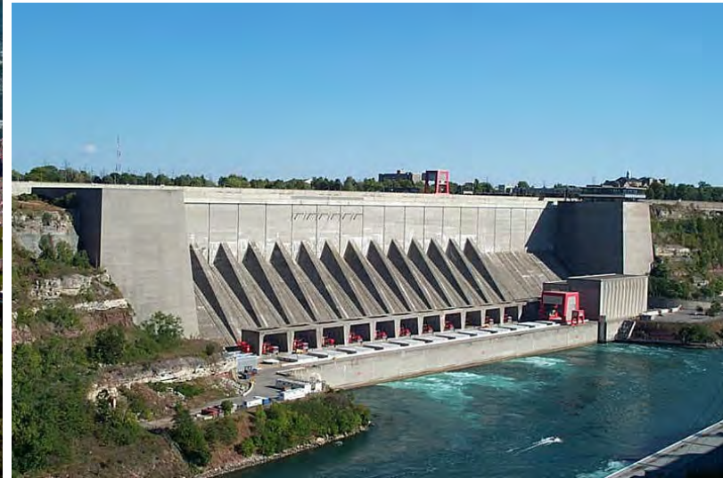
Robert Moses Niagara Power Plant
