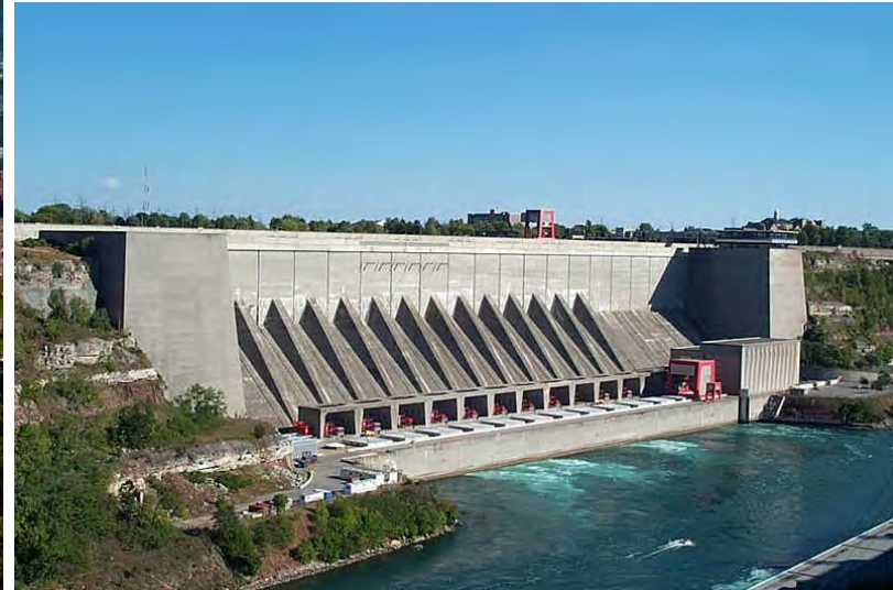
Robert Moses Niagara Power Plant
