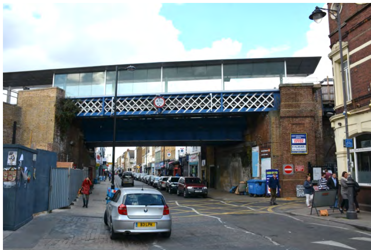
Figure 2: Deptford rail crossing in 2016. John Whiffin’s boyhood house was probably through the arch of the bridge on the right. The original 1840 arches to the right of the bridge still exist, as does the latticework of the bridge itself.
