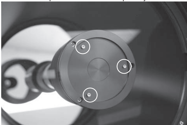
Fig. 15. Collimation screws
