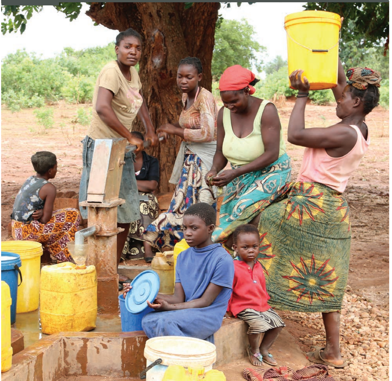
Chileshe Chanda borehole rehabilitation, Hamakumo Village © WaterAid
